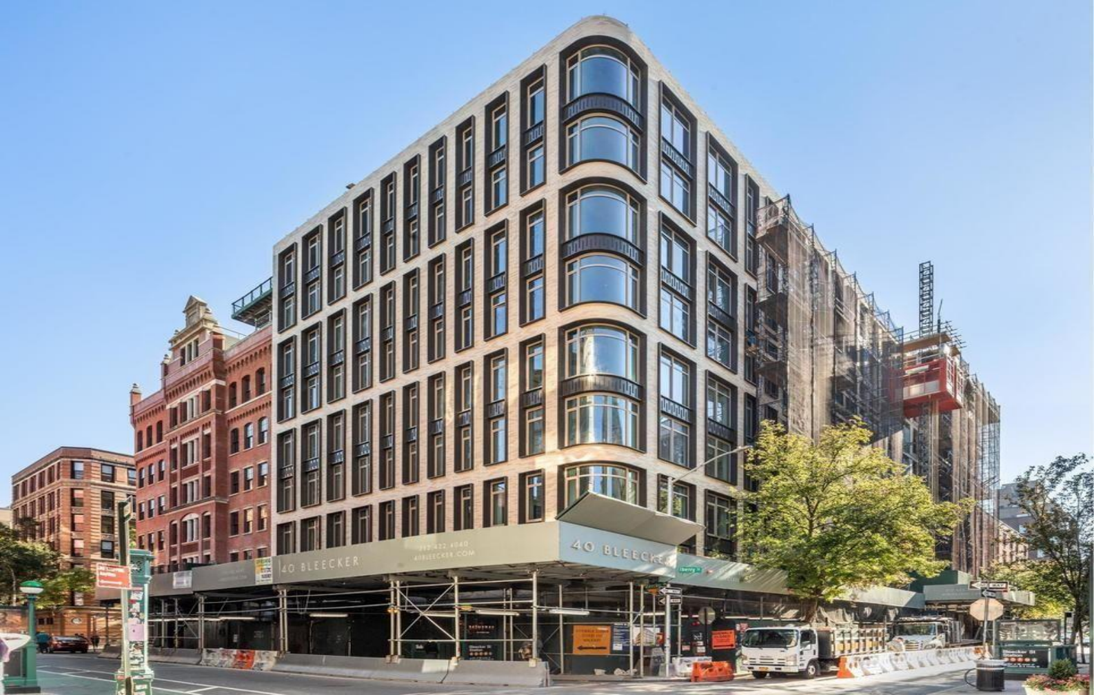
40 BLEEKER STR. NYC NY 66 UNITS 2020 IN PROGRESS KITCHENS
